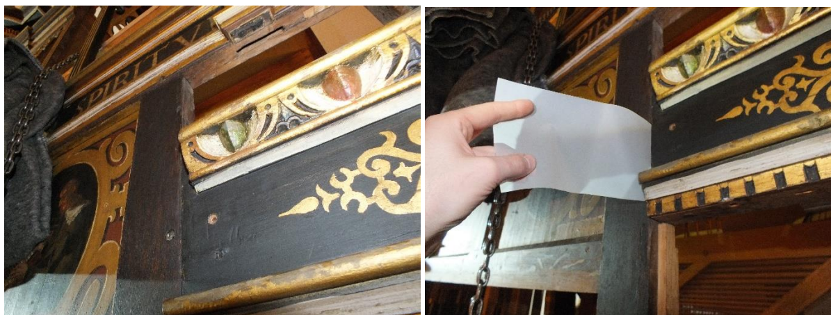
Photo 22: the right joint, seen from outside
