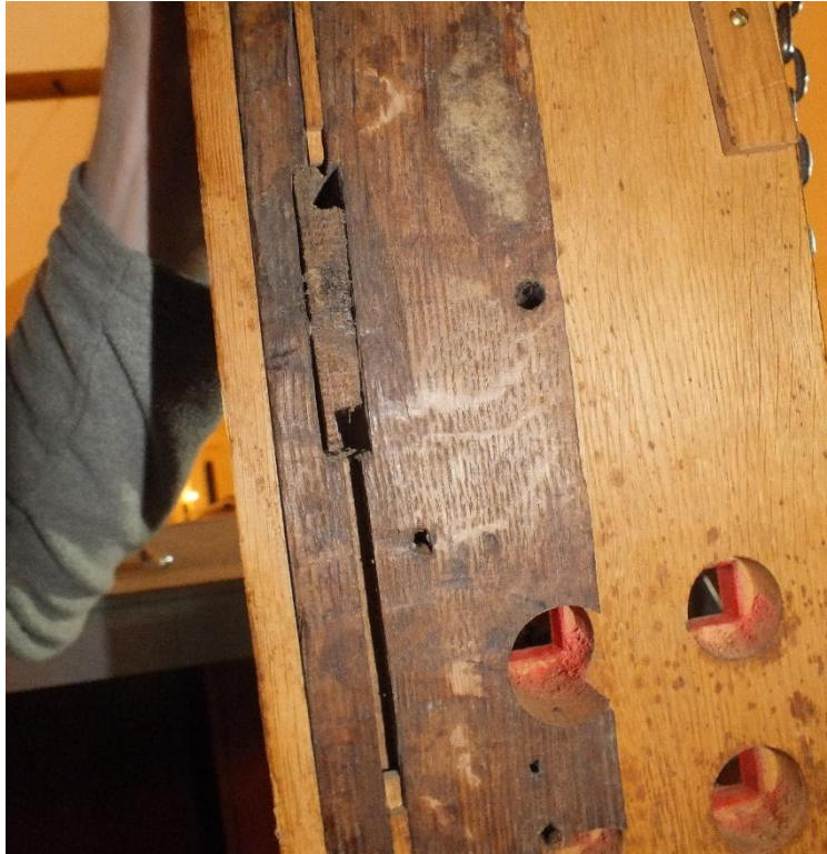
Photo 11: sawn-off tenon from a side rail in the lower case
