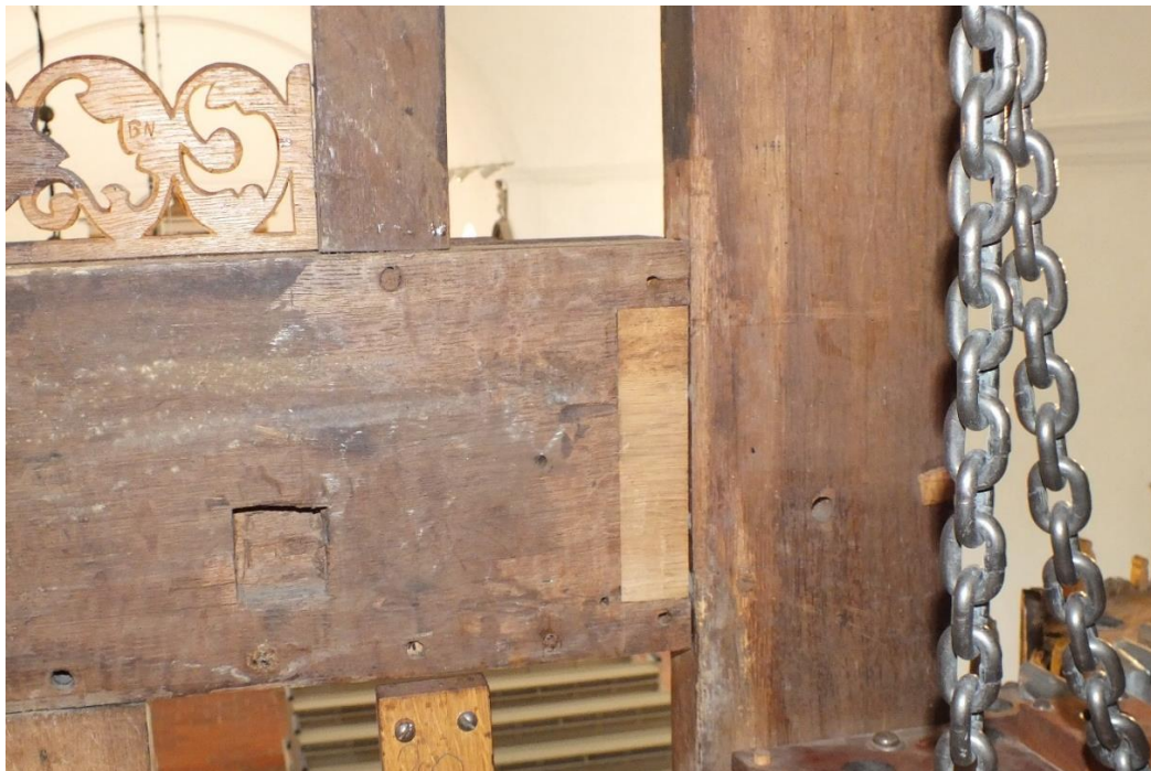
Photo 7: remains of a cornet joint in the rear side of the Brebos impost frame. On the left side an old notch, possibly for a soundboard member, is visible.
