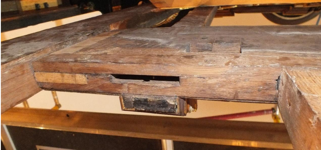
Photo 12: mortises in the underside of the side parts of the impost
