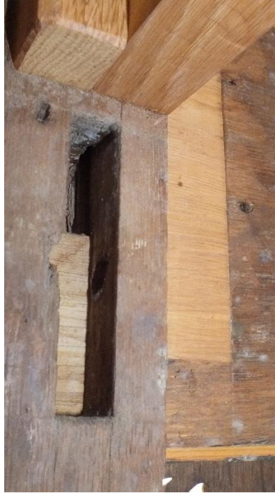
Photo 24: detail of the wood joints on the opposite side
