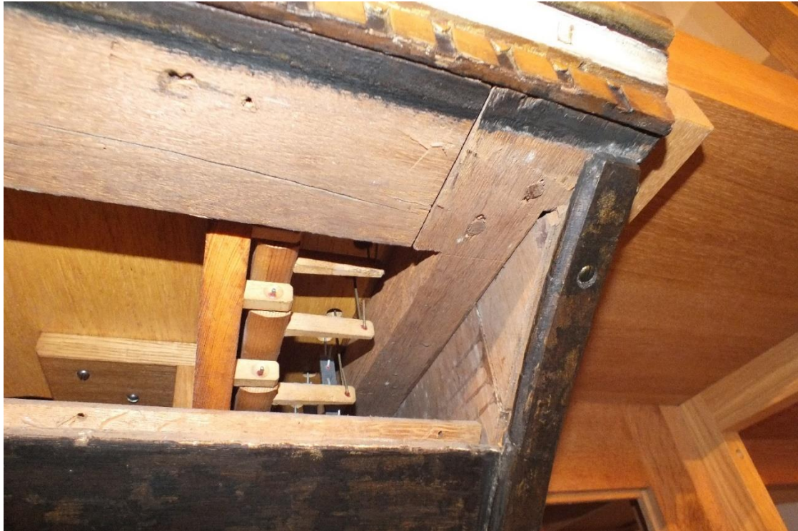
Photo 19: the same frame but showing the side rail tenoned into the rear rail. The rear rail was recently cut out here for the pulldowns of the Frobenius soundboard.
