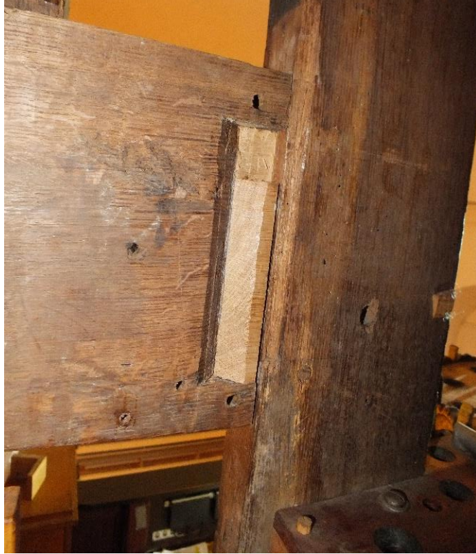
Photo 8: Frobenius material partly chiselled out, revealing the mitred joint
