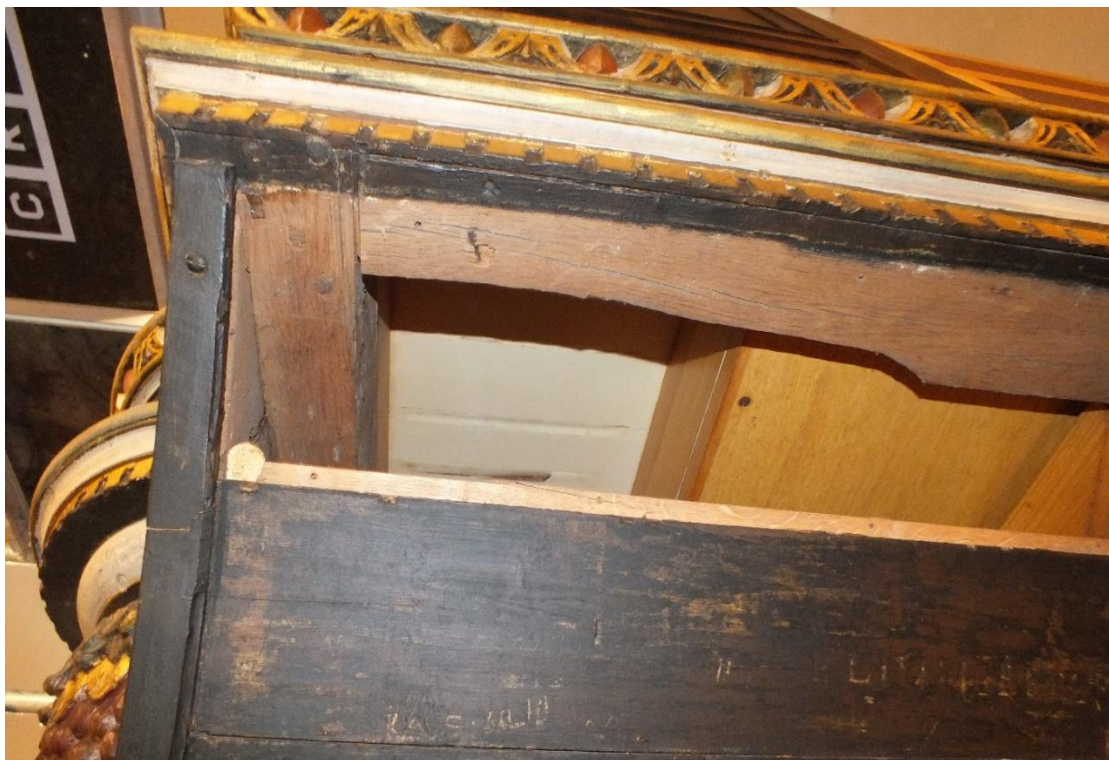
Photo 18: the low frame as seen from below, showing the side rail tenoned into the front rail. There is a very old cutout (perhaps for the last pallet pulldowns at the edge of the soundboard) in the side rail.
