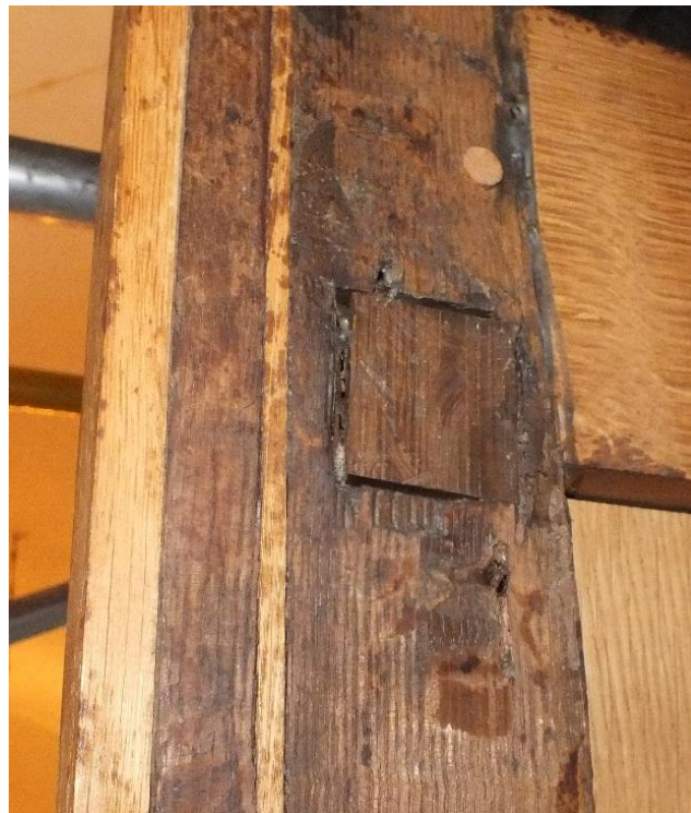
Photo 2: 1850 penetration for stop knob now pieced in.
